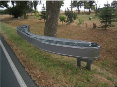
Fig. 16 Denmark: a - an example of fencing the tree growing in the safety zone; b - the lighting pillar made of metal farms
