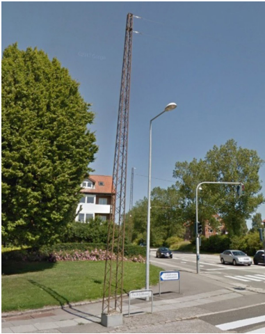
Fig. 16 Denmark: a - an example of fencing the tree growing in the safety zone; b - the lighting pillar made of metal farms
