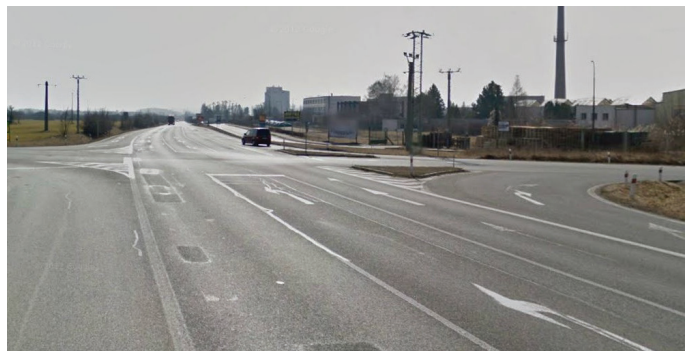
Fig. 8. The view from main road direction to city of Mikulov
