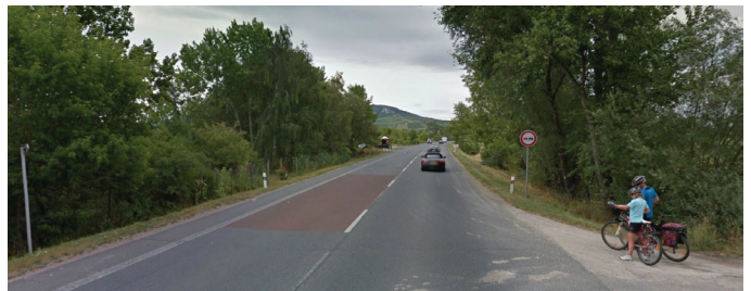
Fig. 8. Location of cycle route crossing with red road marking on the main road
