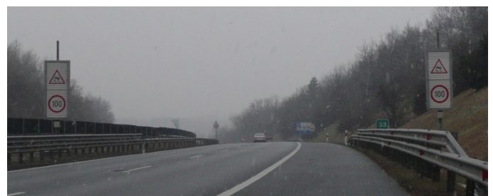
Fig. 3 Prismatic VMS panel during operation [source: MK Zrt.]
